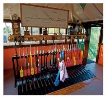
Since 1987 the Friends of Romsey Signal Box have restored the inside of the box to operational order, with various signals and a point connected to some of the levers. Your guide will explain what everything does, and give a simple demonstration of the signal box in operation, inviting you to pull the levers which operate the signals outside.
